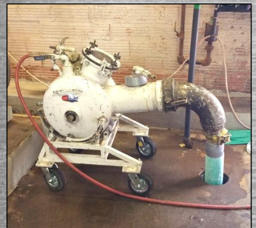
Cured-in-Place-Pipe Lining in Progress
