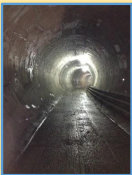
Utility Tunnel access to conduit location
