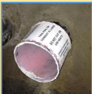
Conduit after Flow-Liner® installation
