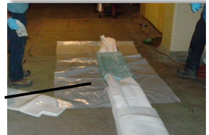
Pipe liner being prepared
