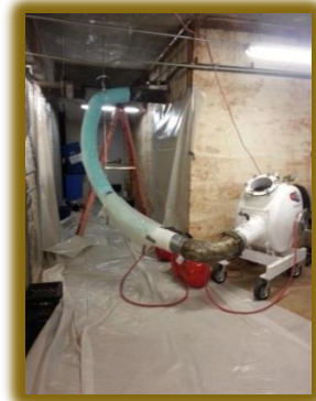
Flow-Liner® Equipment Set-up
