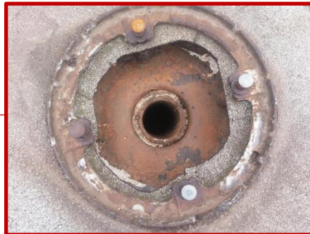
Roof drain body and 3 inch cast iron pipe
