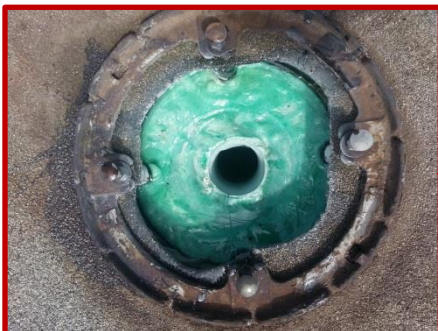
Roof drain body and pipe after Flow-Liner® installed
