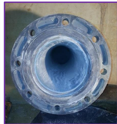
8” main drain pipe after Flow-Liner® installation
