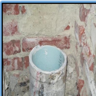
Access point used for Flow-Liner installation
