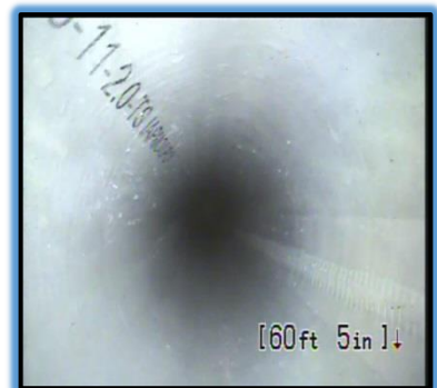
Roof drain after Flow-Liner® Installation
