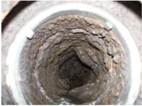
8" Pipe before Flow-Liner® Installation
