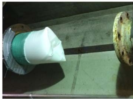
Cured in Place Pipe Lining in Progress
